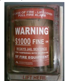
Figure 1 Photo of a pull station cover
