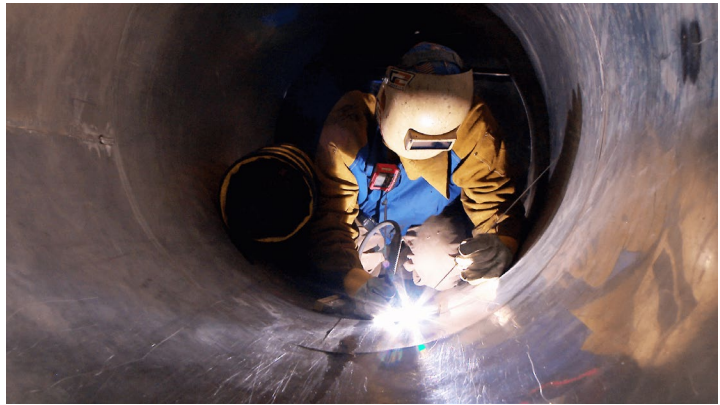
Welding in a tank
