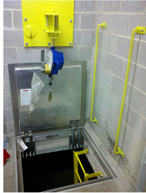
Figure 26: Permanently mounted anchor at confined space entry. SRL is backup fall protection to fixed ladder. (Diversified Fall Protection Co. www.fallprotect.com )
