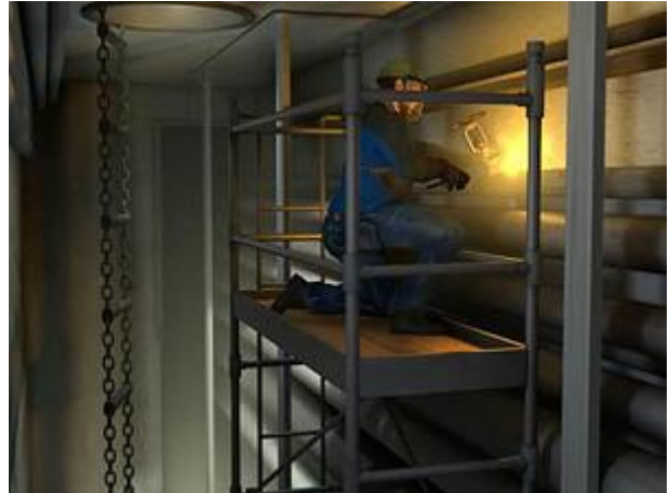
Figure 30: Work from scaffold in confined space www.quadcitysafety.com
