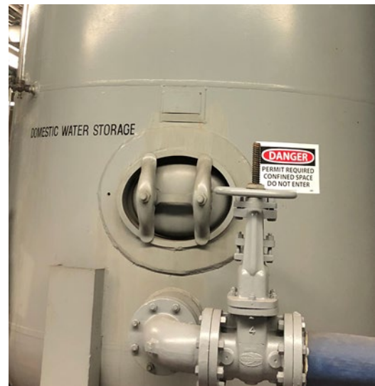
Permit-required confined space: Water storage tank
