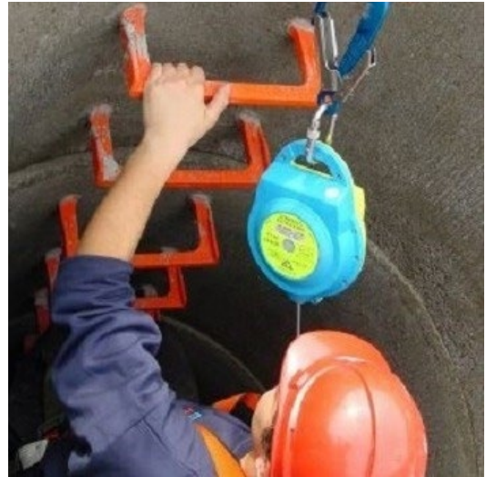
Manhole steps (polypropylene copolymer/steel bar) www.environmental-expert.com/products/iverna-2000-model-manhole-steps
