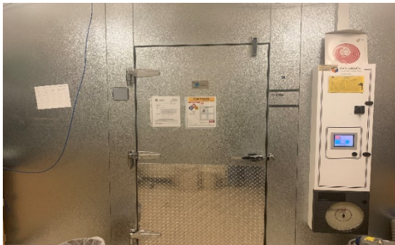
Entry to cold room
