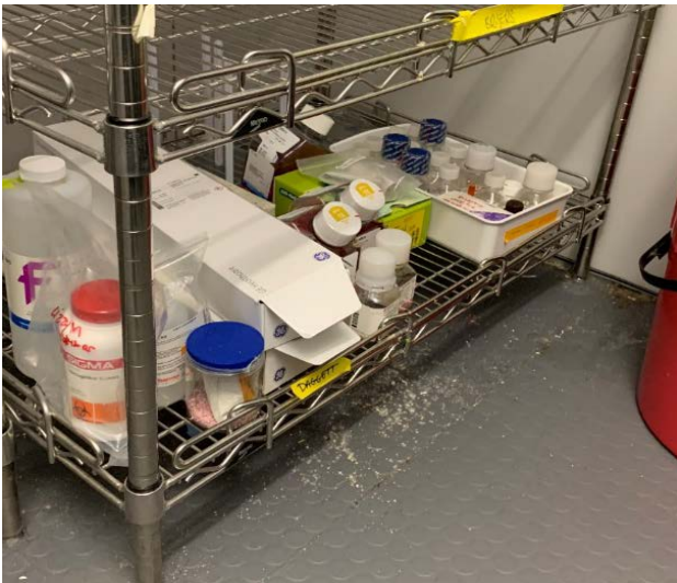
Mold growth on floor in cold room
