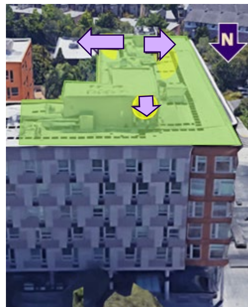
Figure 1: View from the roof.
