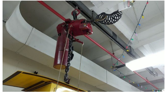
Figure 11: Air - Pneumatic hoist (UW installation)
