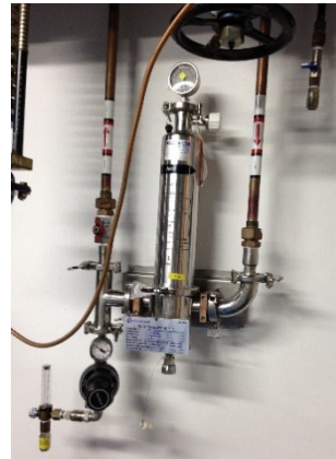
Pneumatic – compressed air with filter
