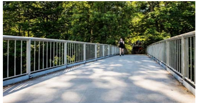
Guardrail system on overpass by E18 parking lot
