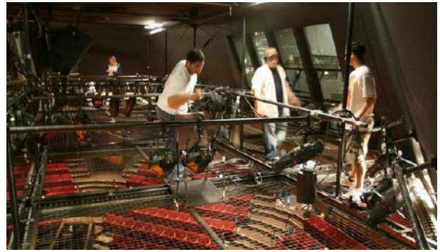
Theater lighting catwalk guardrail system UC Performing Arts Safety Manual
